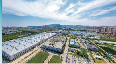
Hisense (Huangdao) Information Industrial Park
