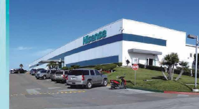
Hisense Mexico Industrial Park
