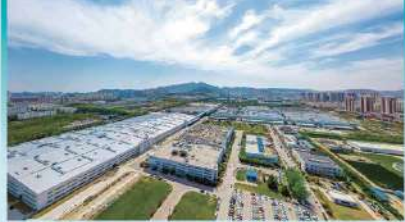
Hisense (Huangdao) Information Industrial Park
