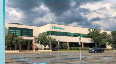
Hisense New Jersey R&D Center, USA
